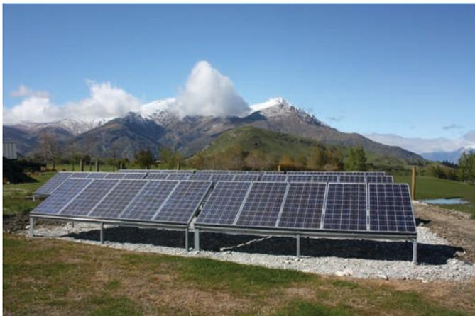
A secluded house in the Queenstown district features one of the most picturesque photovoltaic (PV) installations in New Zealand. The system is rated at an impressive 21.6kWp with the install split between the roof of the house and a ground-mount system.
