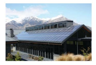
A secluded house in the Queenstown district features one of the most picturesque photovoltaic (PV) installations in New Zealand. The system is rated at an impressive 21.6kWp with the install split between the roof of the house and a ground-mount system. In total 120 Mitsubishi Black Diamond Solar Panels were installed.
