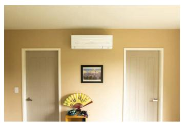
In the master bedroom and two spare rooms, smaller AP Mini units were installed. As a result, only occupied rooms are turned on to heat or cool, ensuring Lucie isn't paying for more energy than is required. When guests stay they have the option to tailor their heating or cooling to the temperature they desire ensuring a more comfortable night's sleep.
