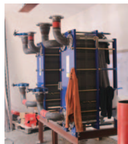
Plate heat exchanger (Field supplied)
