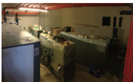
Ground Source Hot Water Heat Pump
