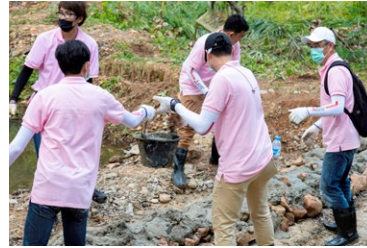
Building a reservoir
